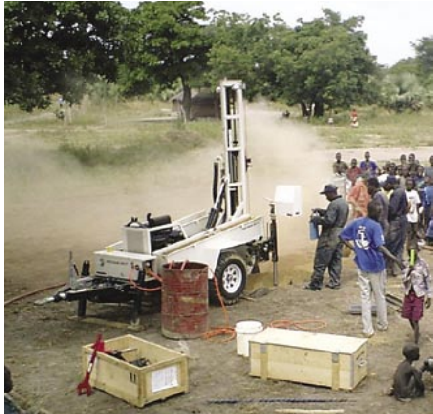
A portable drilling rig with DTH capacity.
