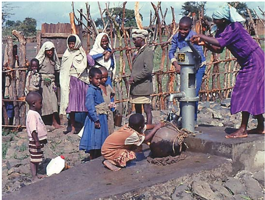
Shallow and medium depth boreholes supply rural water handpumps
